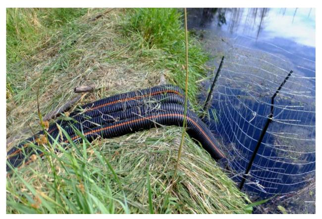
Syphon intake: [4 hoses 5"OD, 0.8m head, ~87 L/s total; my guess, simulating a 200mm ID PVC pipe]
