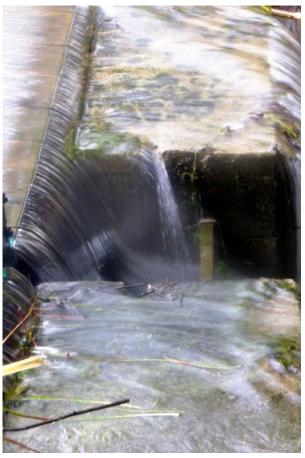
flood, the level 180 mm above the top of the culvert, water extending 15 metres along each side of the path, a rough estimate 85 litres/sec. NE Arm spillway also flooded.
