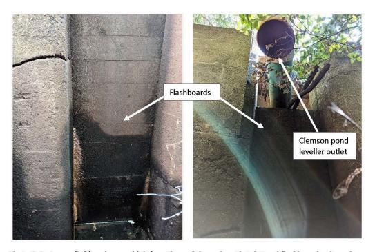
Photo 2.4 Lower (left) and upper (right) portions of the weir outlet slot and flashboards, viewed from the downstream channel. Note cracks in the concrete at several locations (NHC, Sep. 2022).
