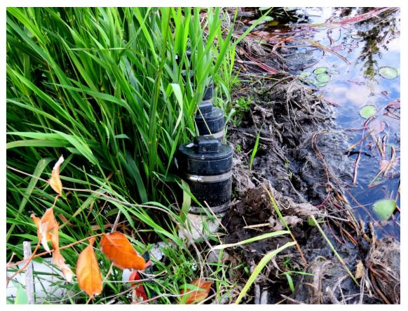
Mud berms now reducing flow around the ends of the dam. Syphon system not functioning and almost buried. No longer an eyesore.
