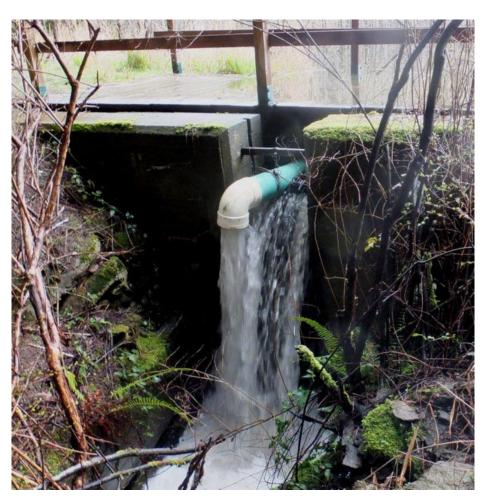
Deck partially flooded as before with a strong flow into the bypass slot along the deck's south side-the deck has become another sill; some flow also on the north side from the bank into a hole leading underneath the deck. Baffle sill +180 mm.
