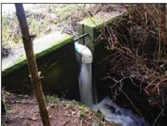
Concrete weir and pond leveler controlling water levels at the outflow of the wetland area on the west boundary of the Coats Marsh RP. (FBER Ltd photo)
