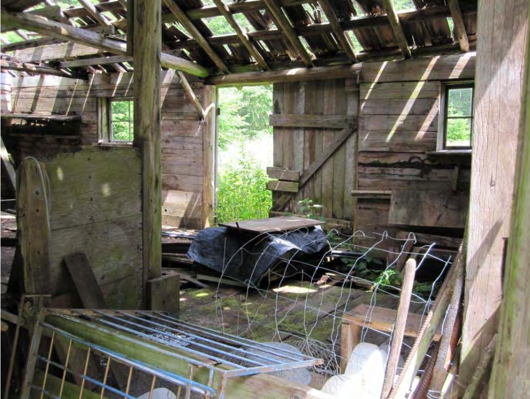
Interior view of Barn.
