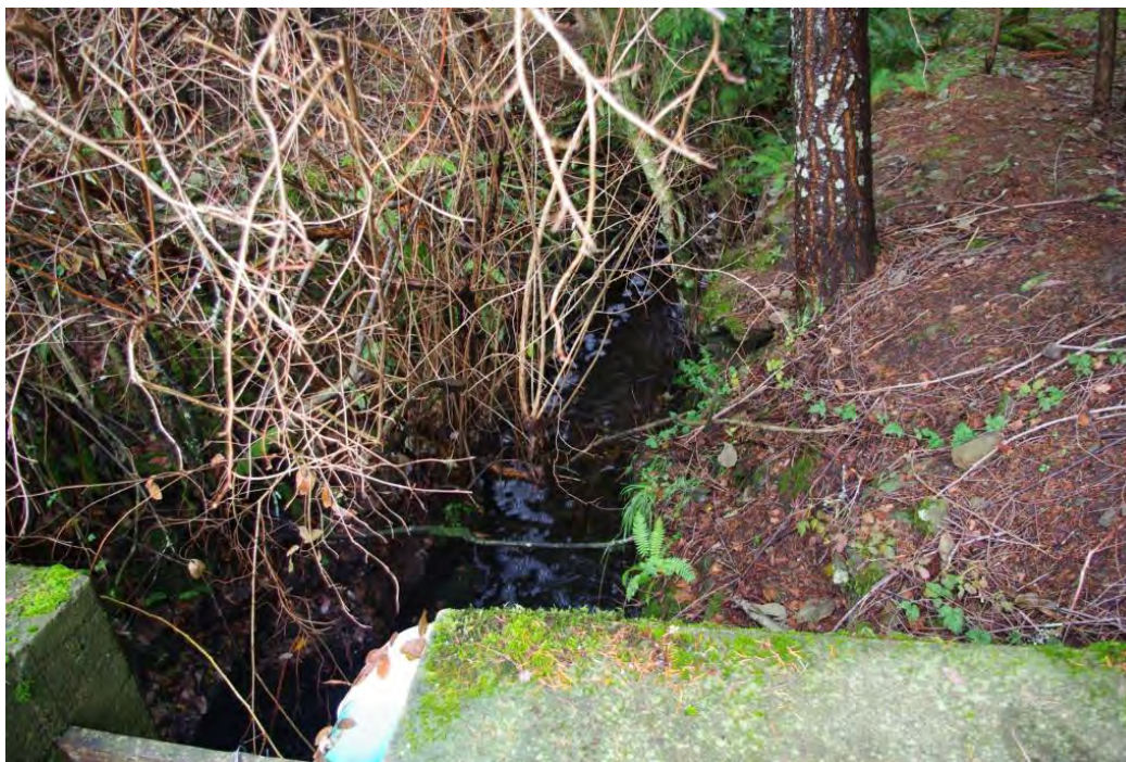
Photograph 10: Water discharge from Coats Marsh looking downstream of the weir.
