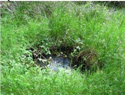
Open surface well at Coasts Caretakers House.
