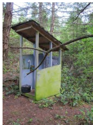
Open Pit Toilet at Coasts Caretakers House
