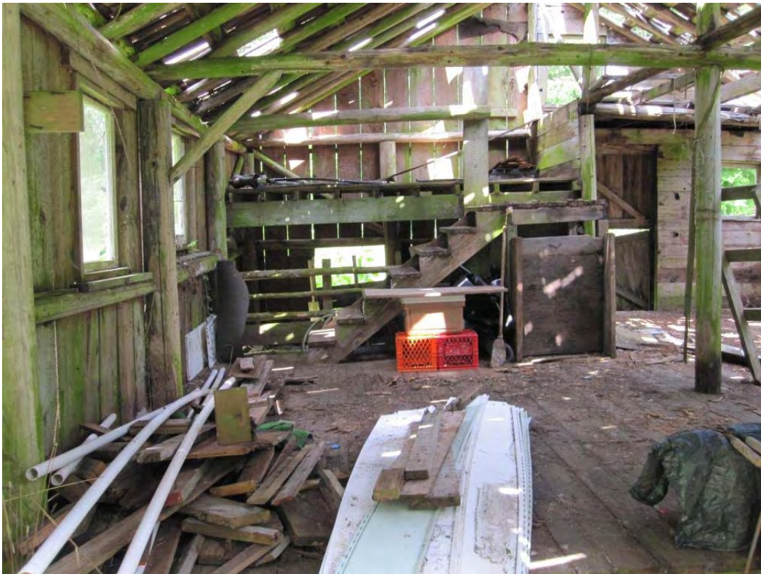
Interior view of barn.
