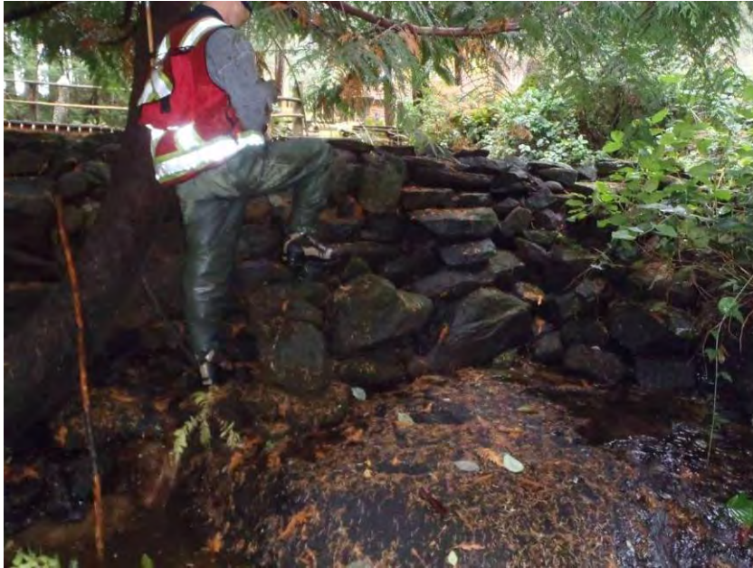
Constructed rock dam located on residential property downstream of Coats Marsh.
