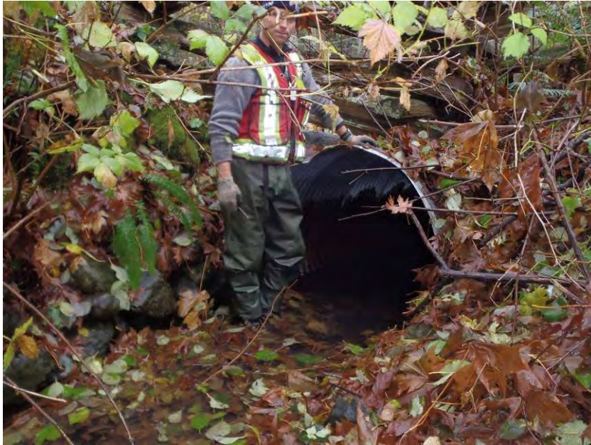
Outflow of the culvert under South Road.
