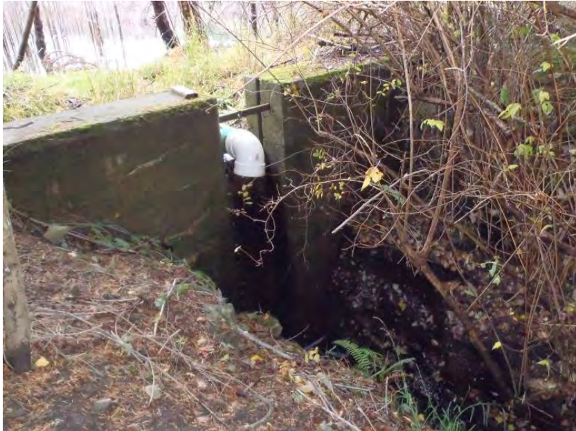
Weir and pond leveler representing the origin of the Coats Marsh outflow stream.
