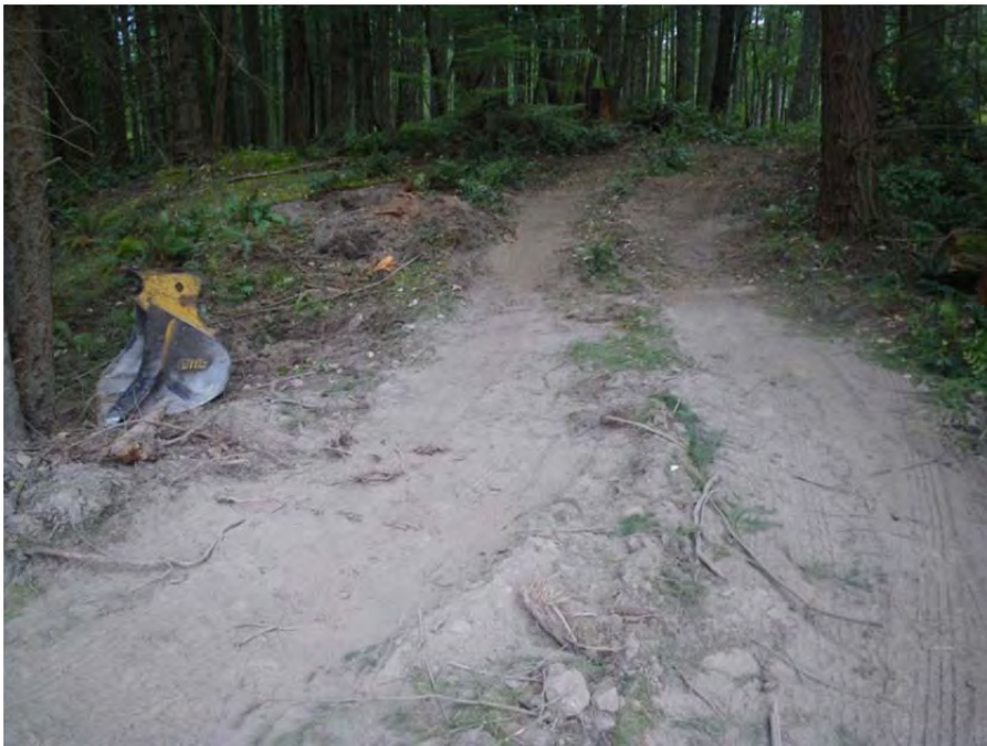
Surface of access road following use by excavator, backhoe and dump truck.
