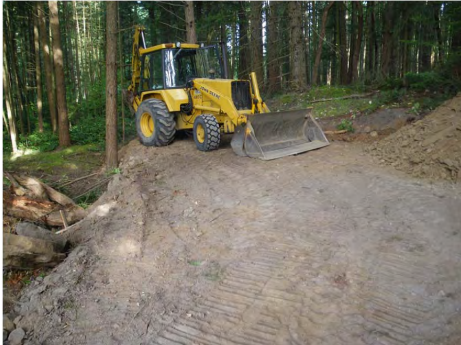
Machine turnaround area at end of access road.
