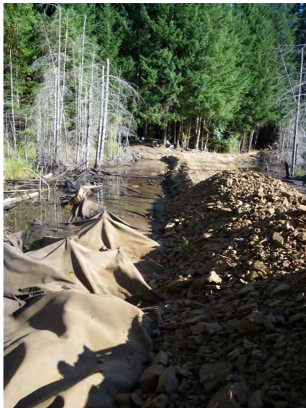
Looking north west over the berm during the construction process.
