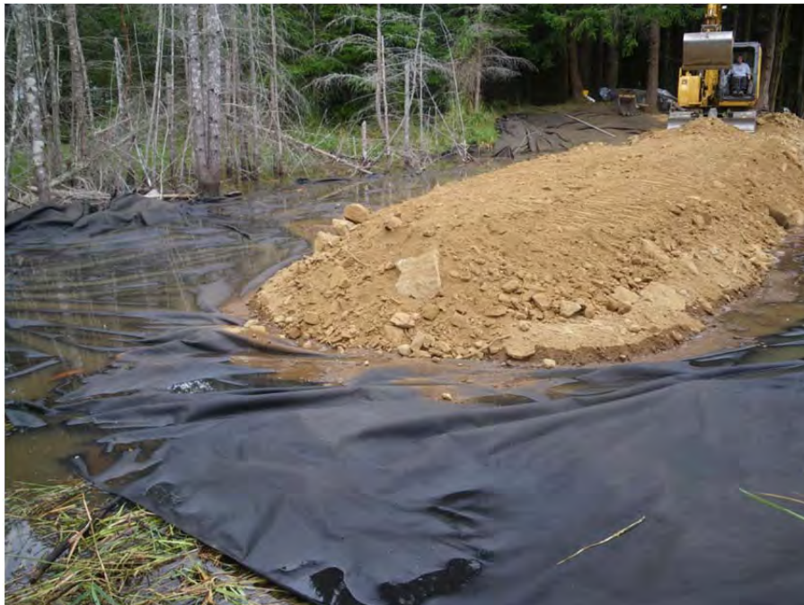
Continuation of fill placement over the geofabric.
