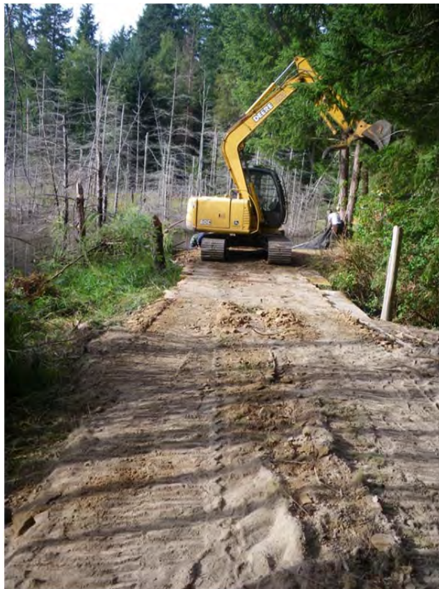
Excavator accessing berm construction area.
