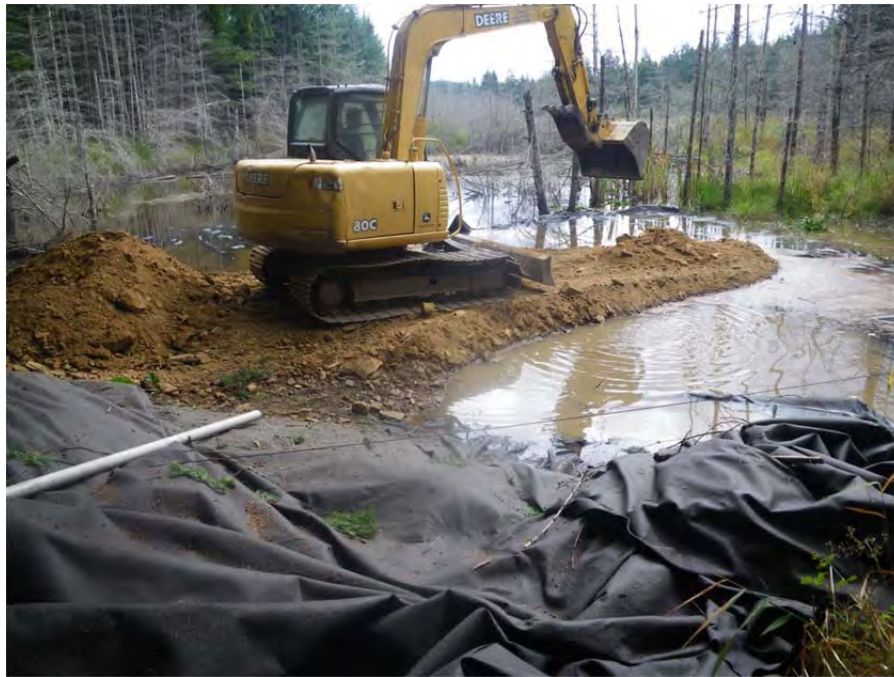
Constructing berm out over the geofabric.
