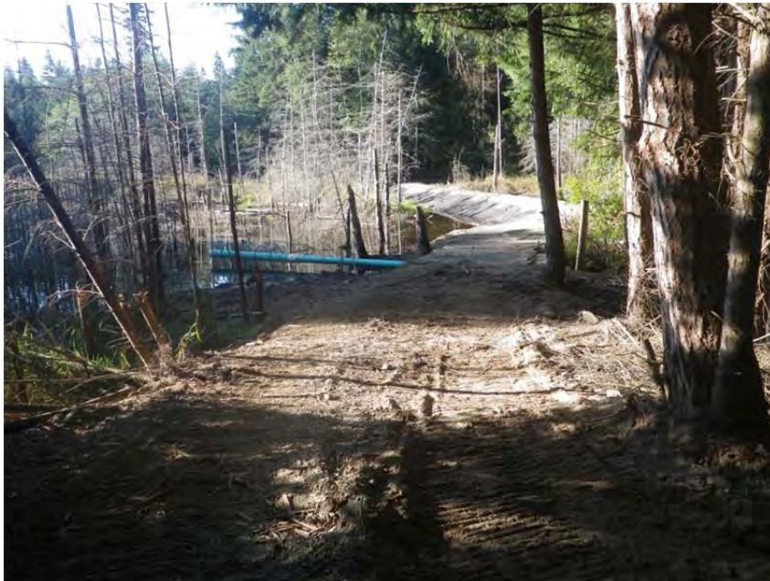
Looking north towards the completed berm, showing the new pond leveler.
