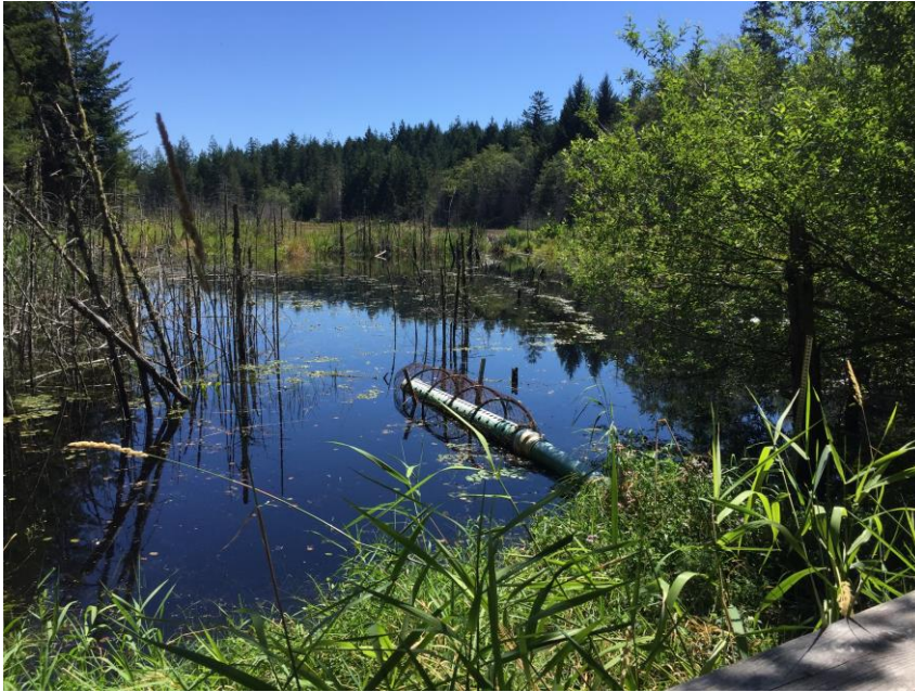
Photo 12. Similar view as the previous photo, showing elevated embayment levels after installation of the draw down siphons on the afternoon of August 4 th , 2021. Flow over the weir, and through the leveler, was initiated following draw-down siphoning over the course of the day.
