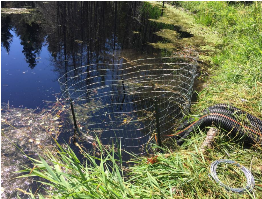
Photo 9. Inlet of temporary draw down siphons (caging is to offer protection from beavers). August 4 th , 2021.
