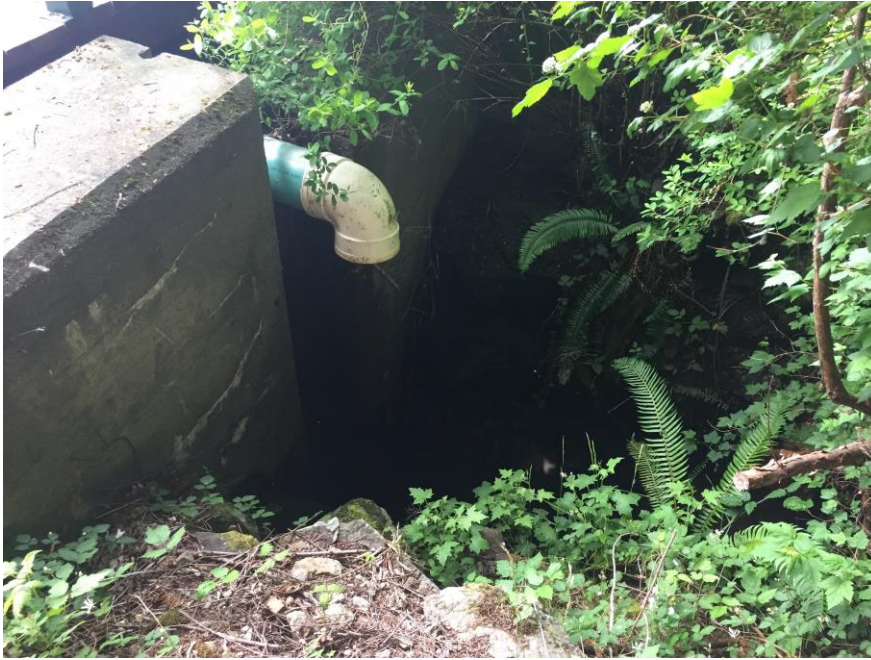
Photo 3. Outlet of the leveling device – May 25 th , 2021. Note lack of flow, which is expected based on time of year.
