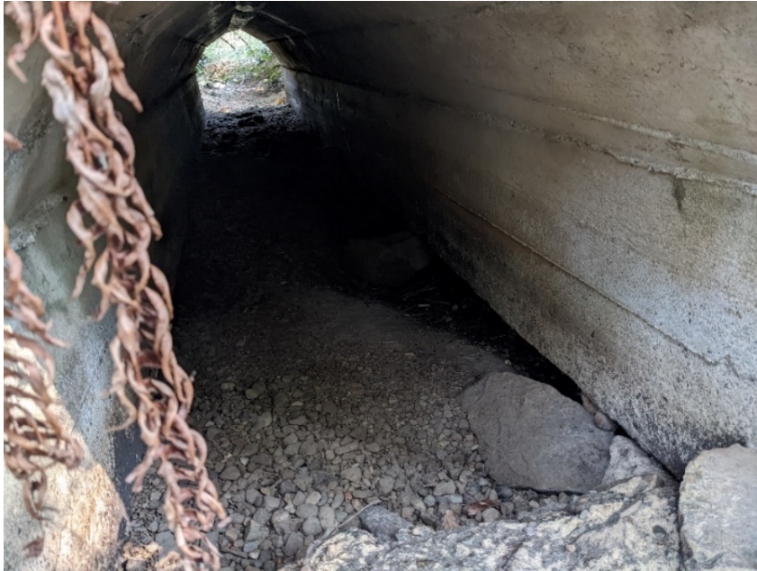
Photo B23 Culvert for Coats Marsh Creek below easement access.
