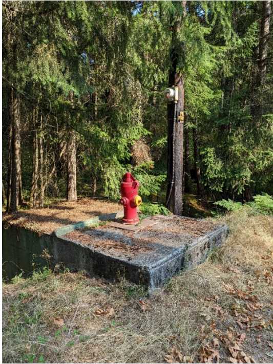
Photo B25 Fire hydrant and pump house located at South Road near Coats Marsh Creek.
