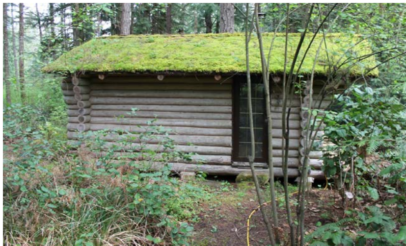
Photo 4.2 Condition of cabin at 1040 Coats Drive (SRM Projects, 2020).
