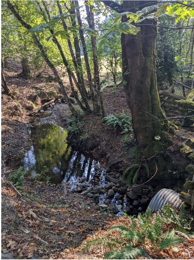
Photo B27 Outlet of South Road culvert crossing. Coats Marsh Creek flows another 200 m through private property before entering Hoggan Lake. Bedrock step feature acting as barrier to most fish passage is downstream of this location within private property.
