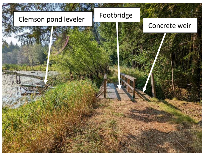
Photo 2.2 Coats Marsh Weir, viewed from the right abutment (NHC, Sep. 2022).
