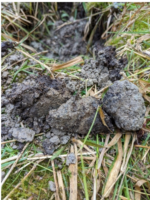
Photo B18 Excavated materials from test pit, representative of conditions for the foundation of the berm.
