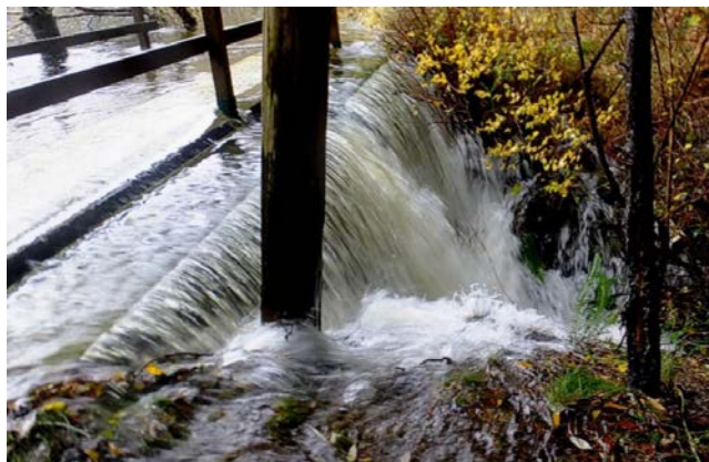
Photo 2.1 Overtopping flow at Coats Marsh Weir during the November 15, 2021 atmospheric river event (Doe, 2021).
