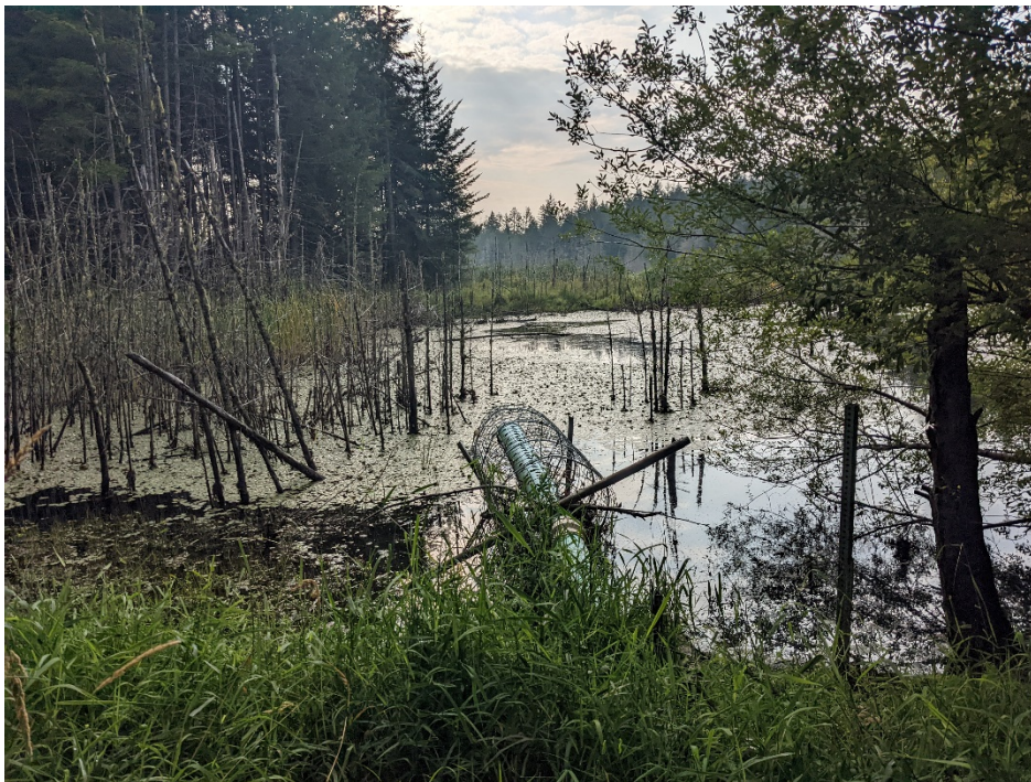
Photo B8 View from weir toward beaver dam, with caged inlet pipe.
