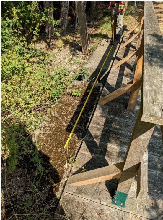
Photo B10 Top view of weir.
