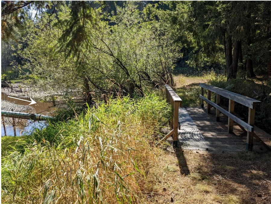
Photo B9 Pedestrian footbridge and weir, looking toward berm (14 Sept 2023).
