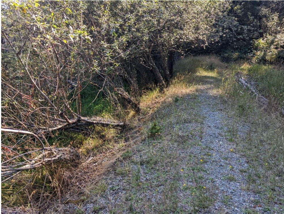
Photo B15 Berm, willows are wrapped in wire to prevent beavers from eating them (22 Sept 2023).
