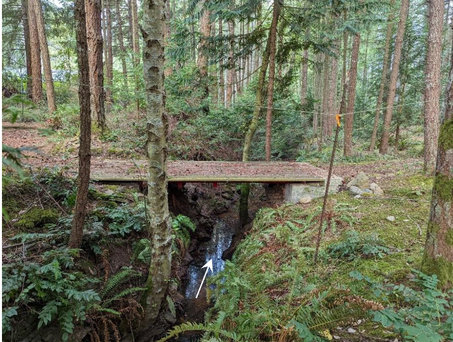
Photo B21 View toward private property where Coats Marsh Creek enters 1040 Coats Drive. Private wooden footbridge. Marker indicates property line (14 Sept 2023).
