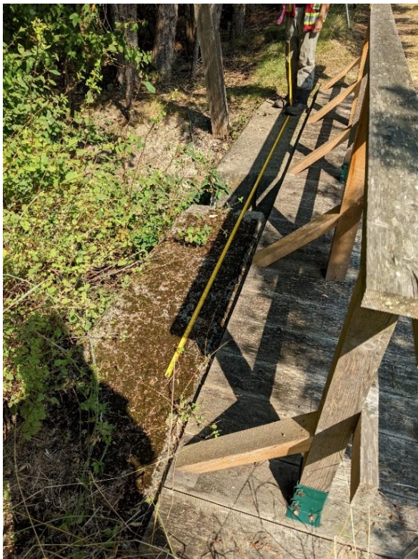
Photo B10 Top view of weir (14 Sept 2023).
