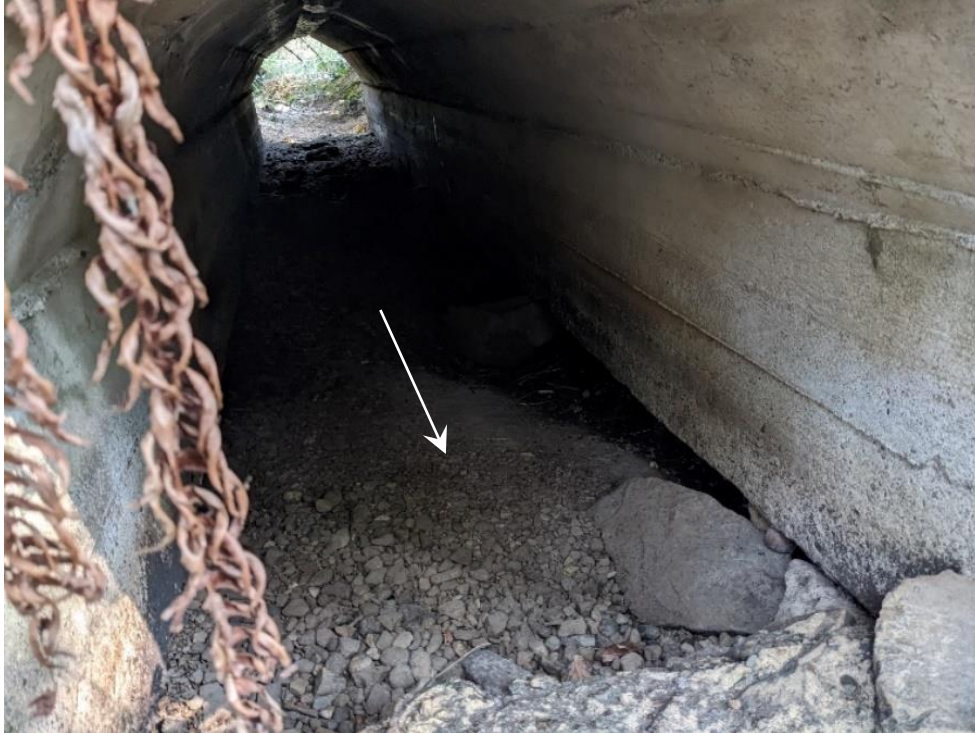
Photo B23 Culvert for Coats Marsh Creek below easement access (14 Sept 2023).
