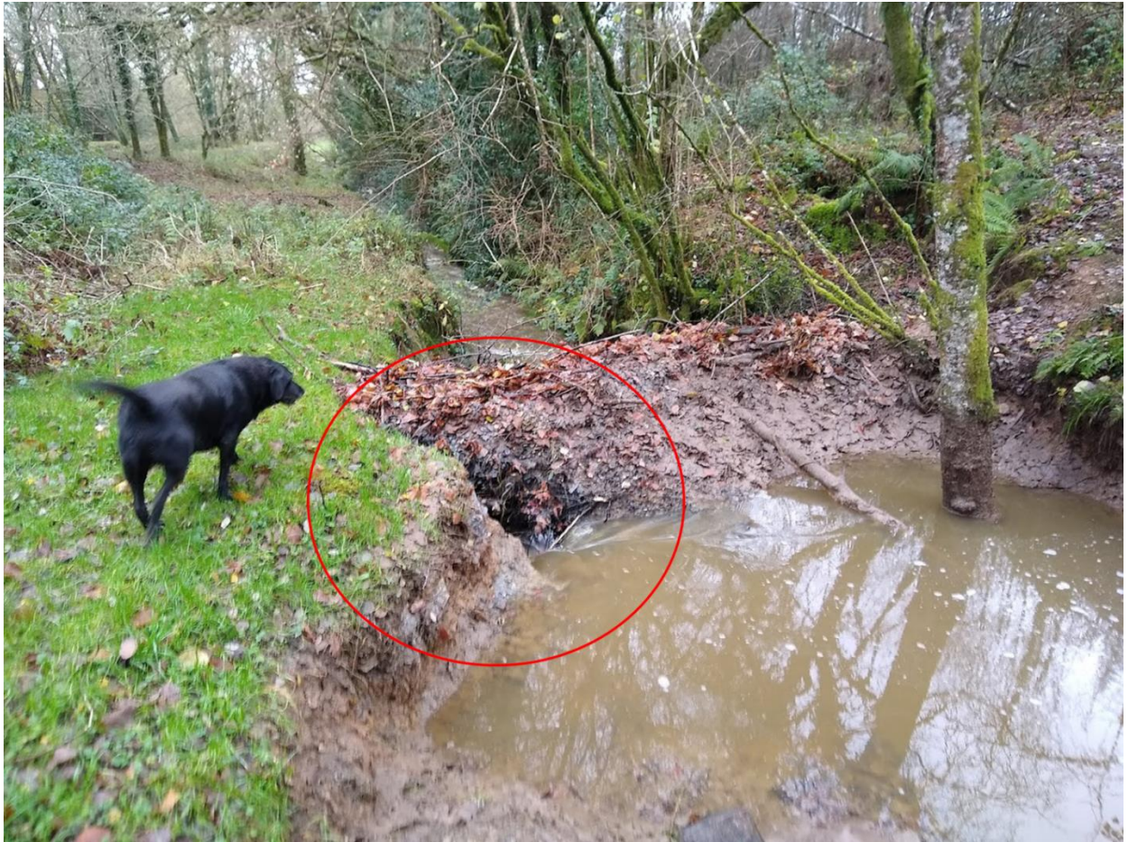
Figure 4. Breach and reduction in water storage in dam on 2 nd order channel
