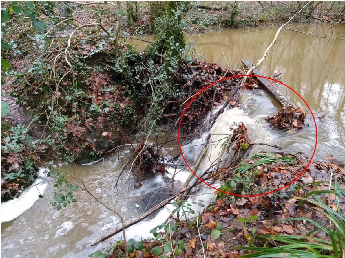
Figure 3. Breach and overtopping of a dam in 2 nd order channel
