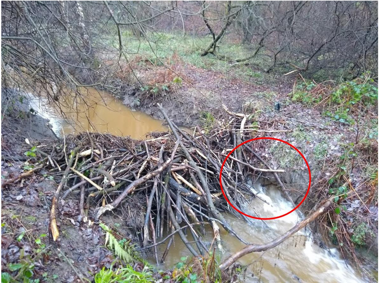
Figure 2. Breach in bottom of a dam on 3 rd order channel
