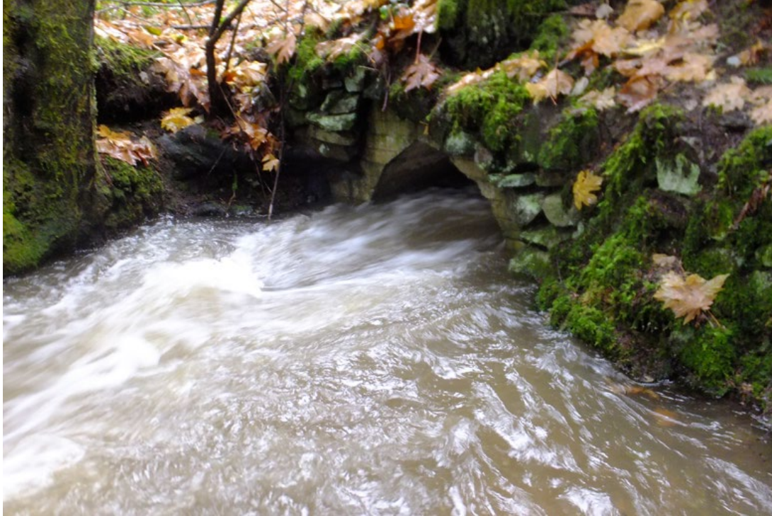
Coats Marsh Creek culvert outlet at the Marsh Nov. 15, 2021
