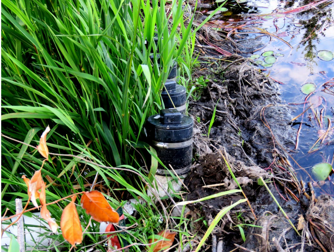
Mud berms now reducing flow around the ends of the dam. Syphon system not functioning and almost buried. No longer an eyesore.
