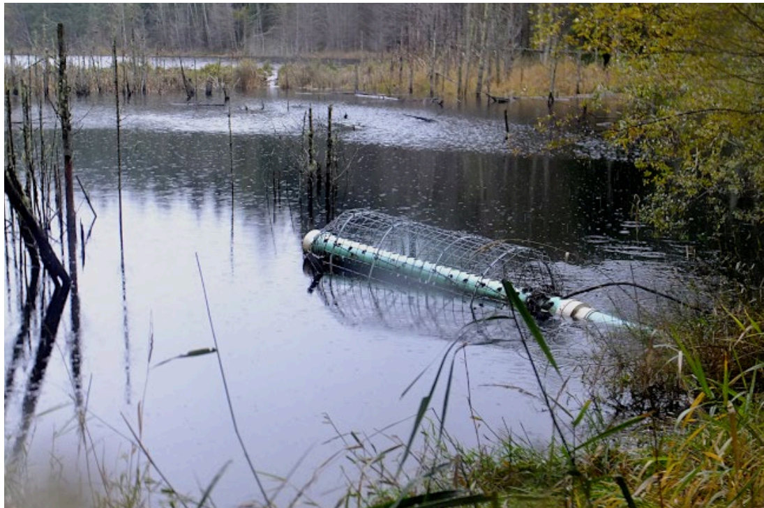
Above: The largest natural spillway in the main beaver dam. Used by the beaver both to reduce overflow and to move back and forth across the dam. The syphon system seen here on the left of the spillway is hidden in vegetation. Below: the pond leveller currently doing its job.
