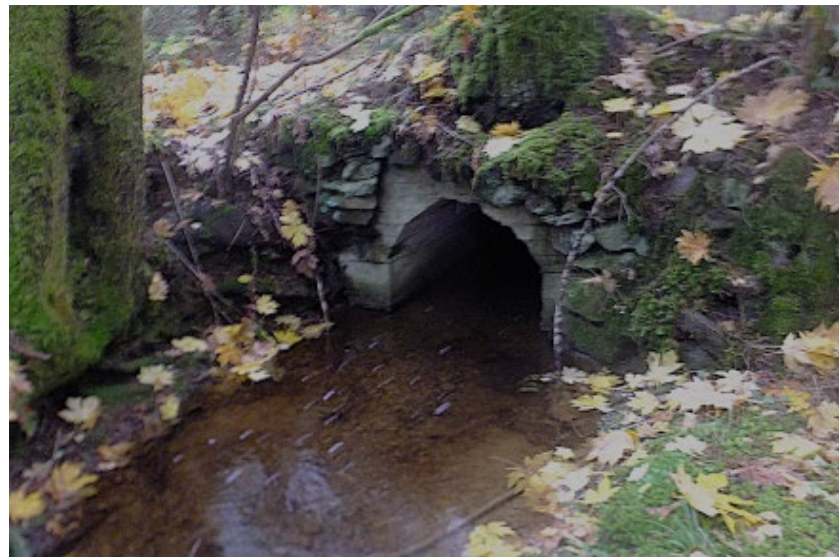
Below: Coats Marsh Creek flowing modestly at the culvert under the Marsh Trail.
