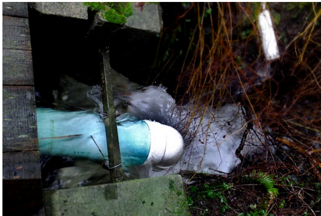
Discharge into Coats Marsh Creek. Rather more than the submerged pond leveller can handle (hard to see in the photo, but the level of water over the sill is higher than the top of the leveller).
