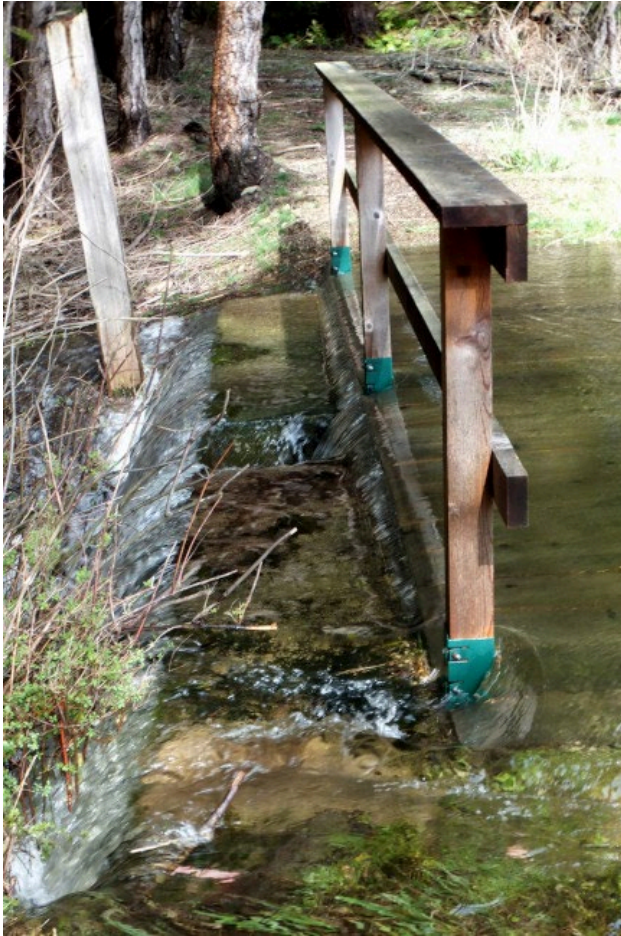
Left: View from the SW corner.
