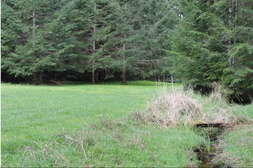
77. Spill channel looing D/S toward 1034 Coats Drive residential property foot bridge 5
