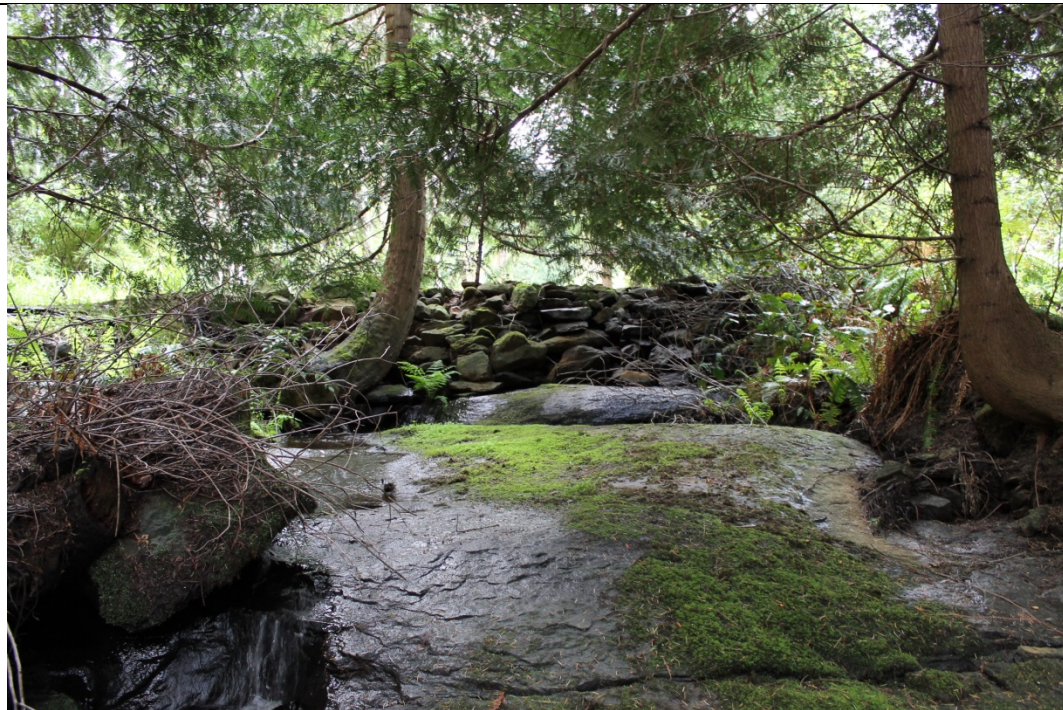
60. Close-up of rock dam in photo 59
