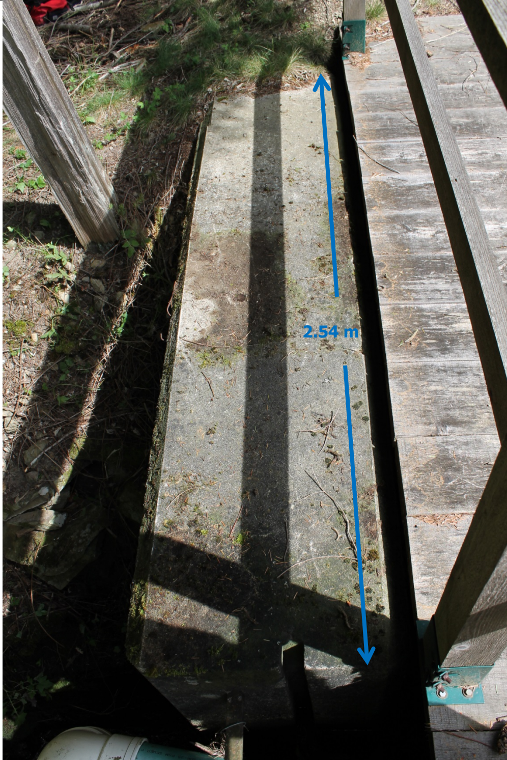
21. Close-up of right concrete weir crest viewed from spillway
