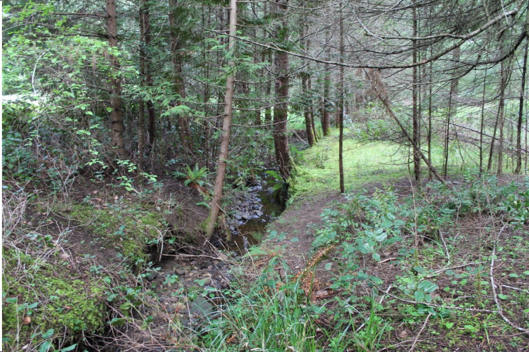
73. Spillway channel looking D/S at foot of 1040 Coats Drive cont'd
