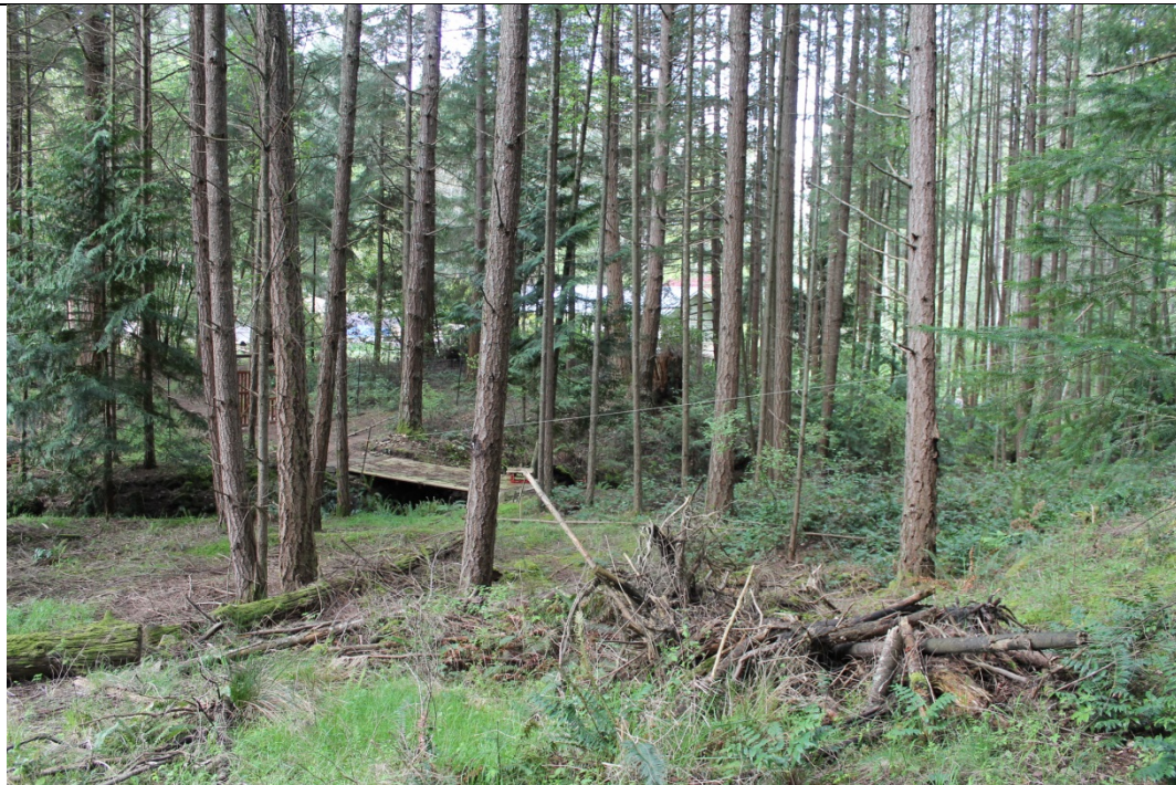
41. Spill path above blasted channel is broad and gently slopes D/S. Trees and bushes will impede overflow.
