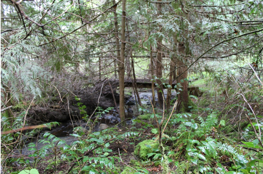
65. Looking D/S at 1040 Coats Drive residential property foot bridge 4
