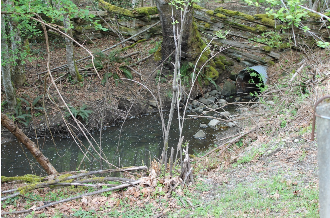
87. Close-up of D/S end of South Road crossing culvert
