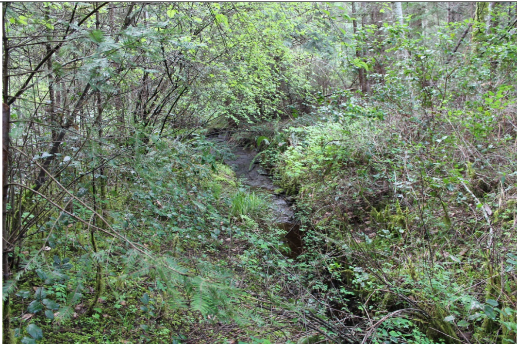
72. Spillway channel at foot of 1040 Coats Drive residential property looking D/S
