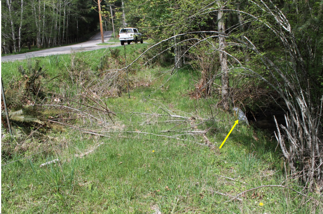
85. View of culvert in photo 84 (yellow arrow) showing South Road crossing
