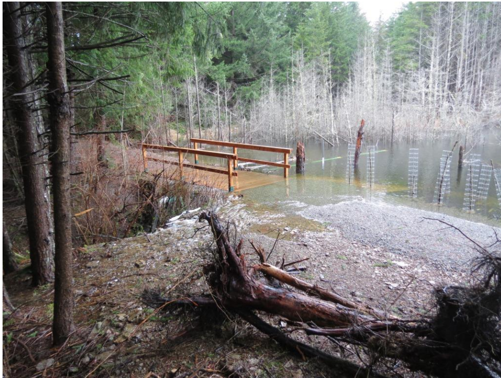
Figure 2-1: Overflow at Coats Marsh weir March 6, 2014
