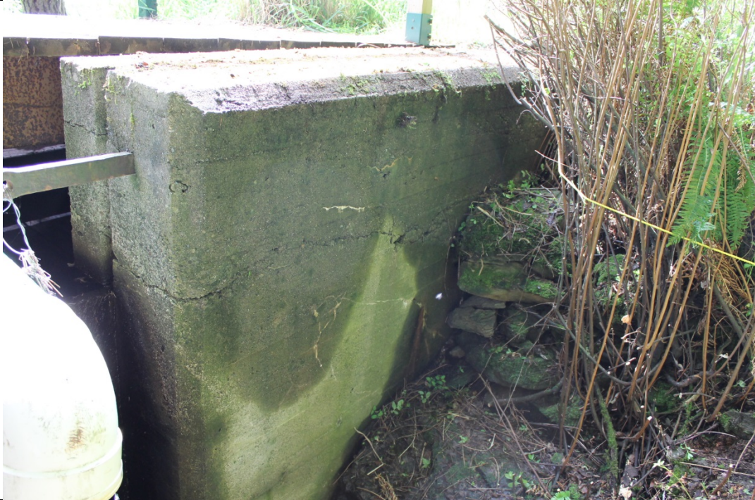
35. D/S face of concrete weir looking toward left abutment
