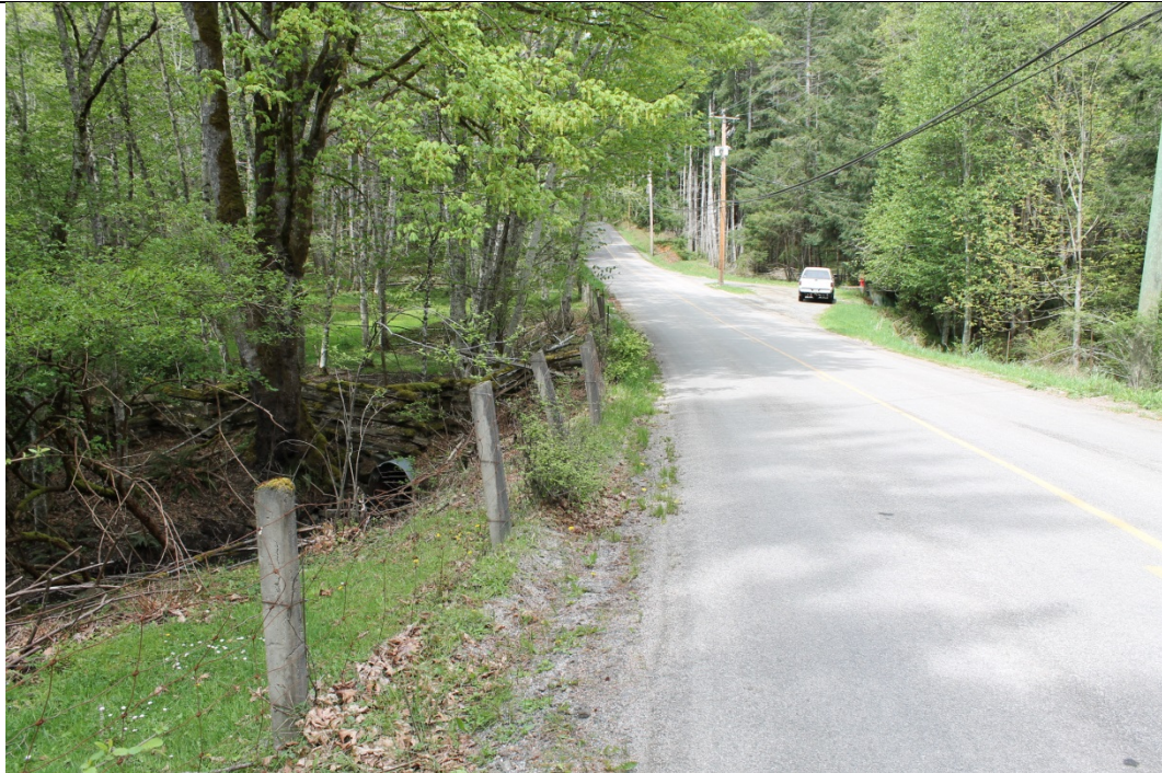
86. D/S end of South Road crossing culvert – culvert crosses at dip in road
