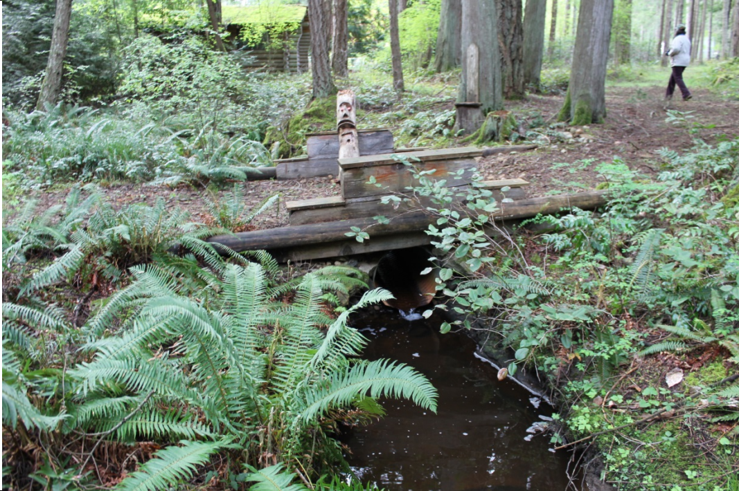
63. Looking U/S over bridge 3
