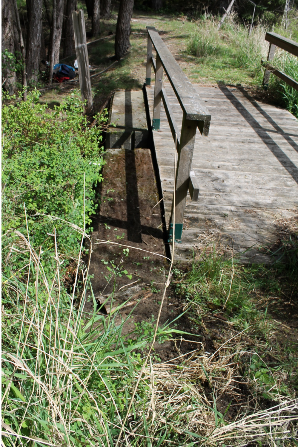
20. Concrete weir crest viewed from left abutment (crest measured to be level)
