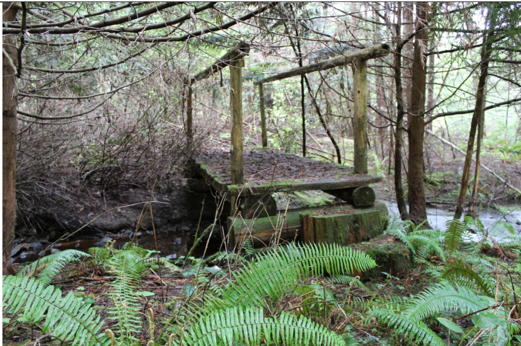
66. Looking from right bank to left bank over foot bridge 4
