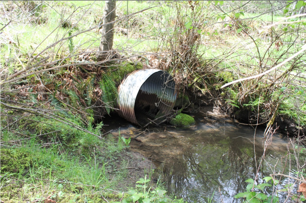
84. 1.22 m dia. Coats Marsh Creek culvert crossing under South Road
