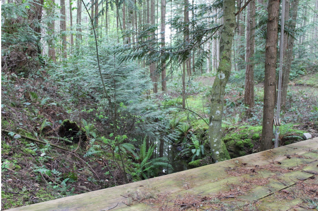
45. Spill channel (aka Coats Marsh Creek) looking D/S from bridge 1
