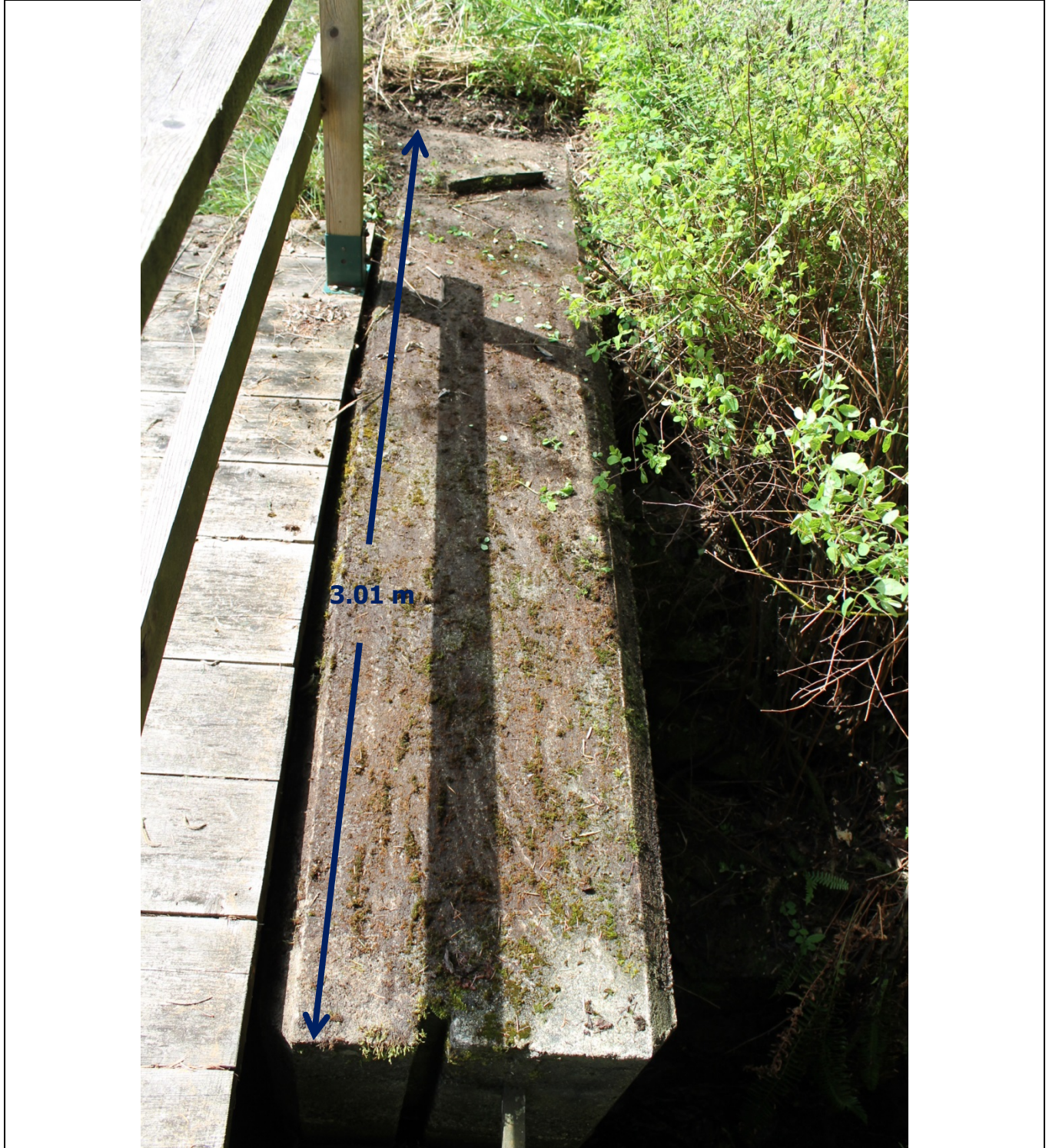
24. Close-up of left concrete weir crest viewed from spillway
