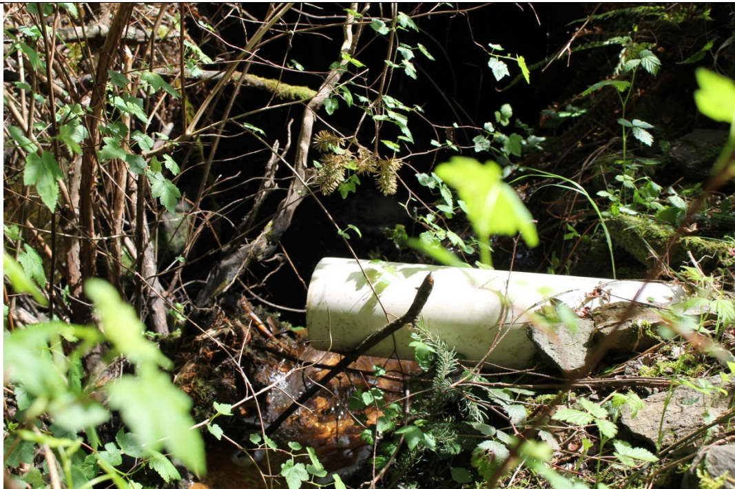
30. Close-up of white dyke downstream drain pipe showing clear water flow
