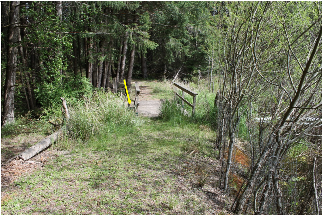
18. Weir crest (yellow arrow) viewed from left abutment side
