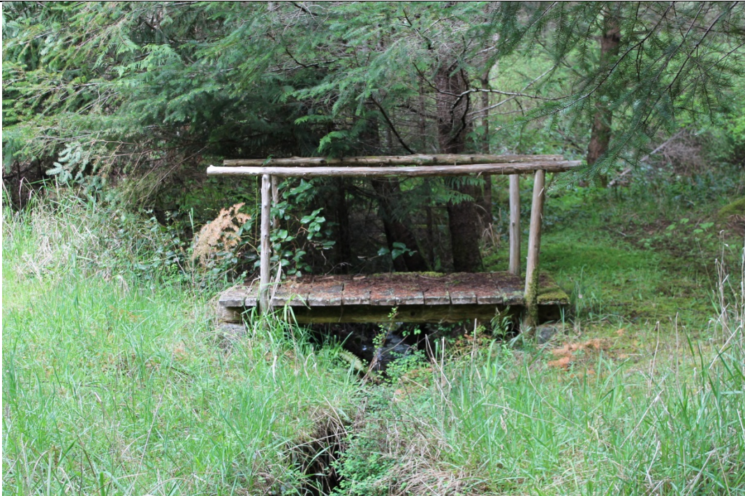
80. Spill channel looking D/S toward 1034 Coats Drive residential property foot bridge 6
