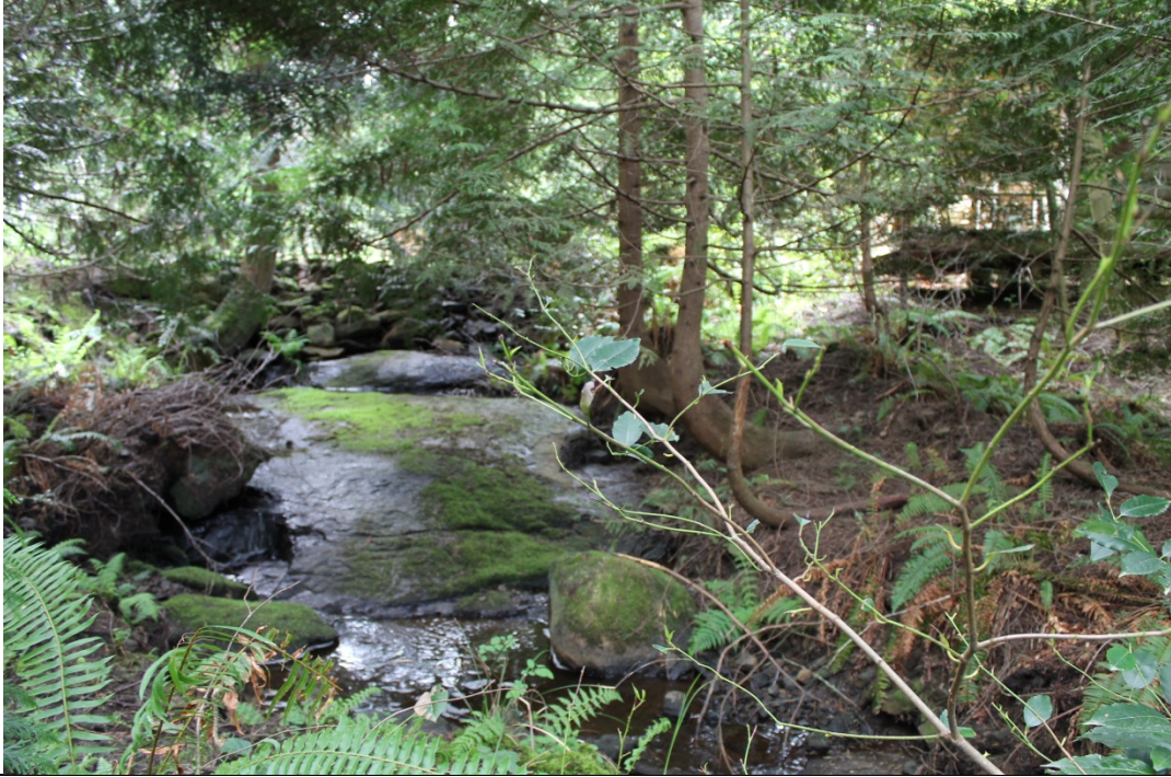
59. Looking U/S at hand placed rock dam near recreational cabin
