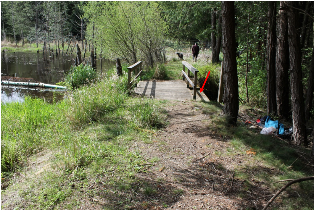
16. Weir crest (red arrow) viewed from right abutment side
