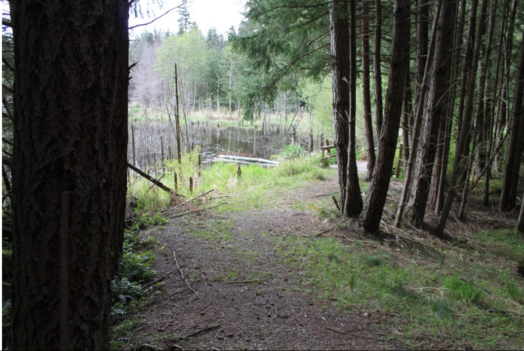
15. Weir crest approach viewed from right abutment side
