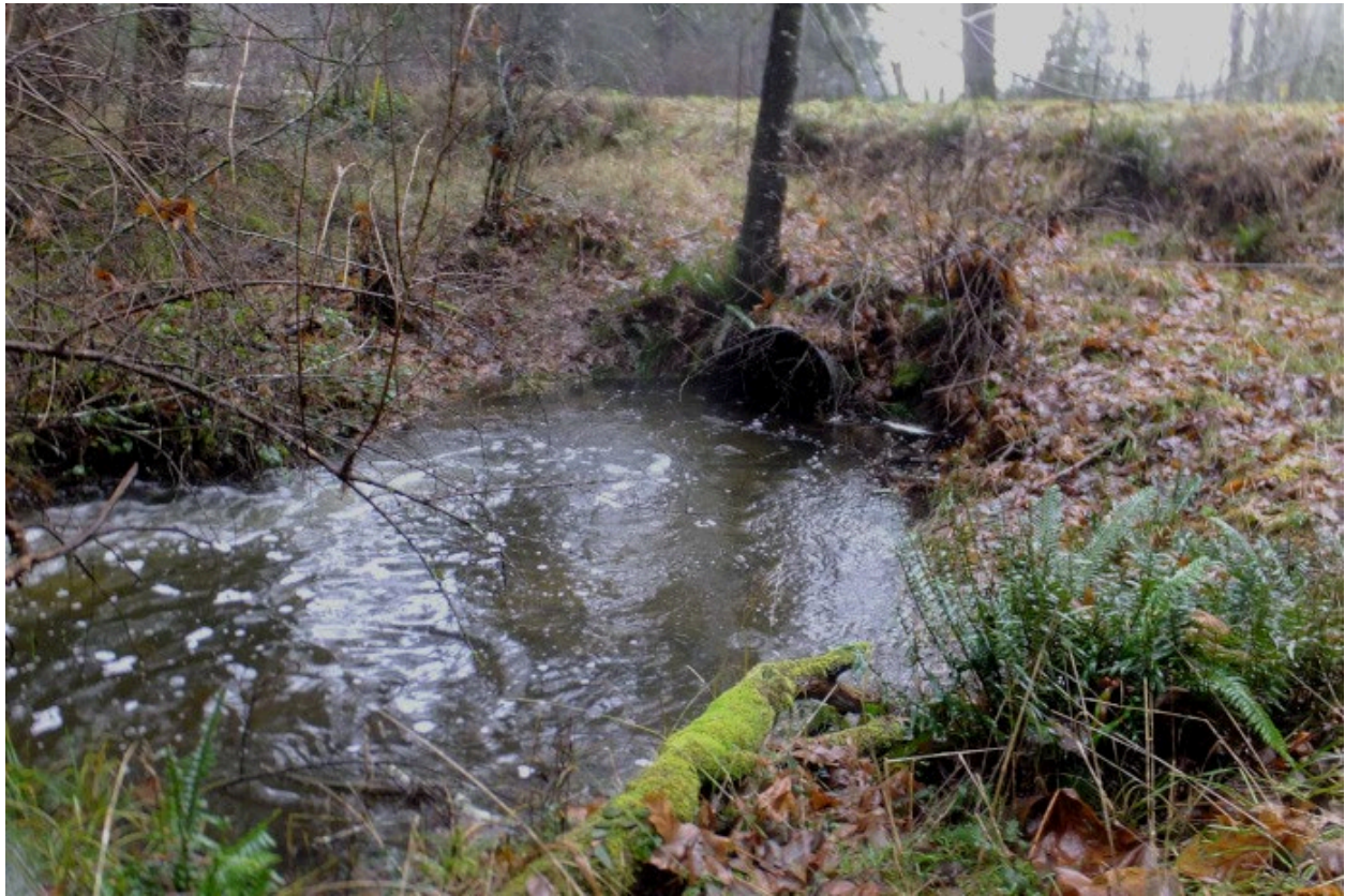
Upper Coats Marsh Creek approaching the culvert under South Road on the upstream (NE) side. No obvious external obstruction to the culvert but the water velocity through it is high.
